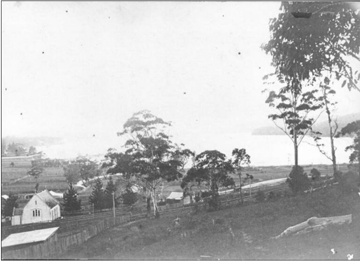
View of the original site of "Our Lady of the Rosary" overlooking Brisbane Water in Donnison St, Gosford current location of NSW Workcover offices.
